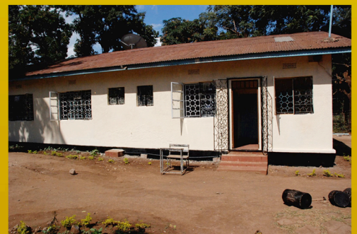
REPAIRED AND PAINTED ENTIRE FACILITY
