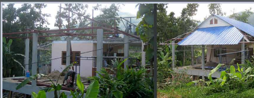
OLD KITCHEN WITH NEW FRAME FOR EXPANSION
