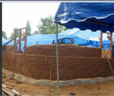
MUD COB CONSTRUCTION
